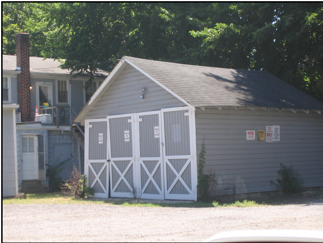
Photo: Garage, northeast corner, looking southwest.
